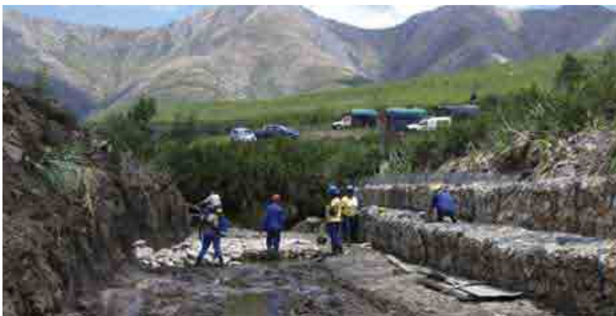
Building gabions to restore a degraded wetland
