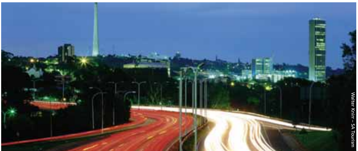
The city of Johannesburg, Gauteng province
