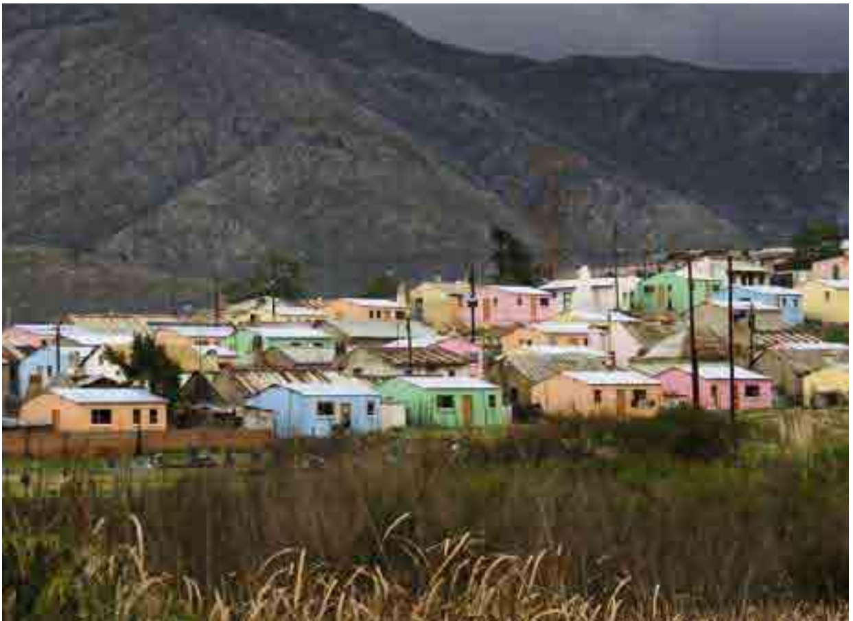
Low-cost housing development, Oudtshoorn, Western Cape
