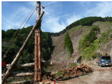
Figure 6: Lumber transport and a forestry road
