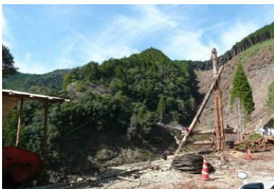
Figure 5: Logging site for cedar and cypress
